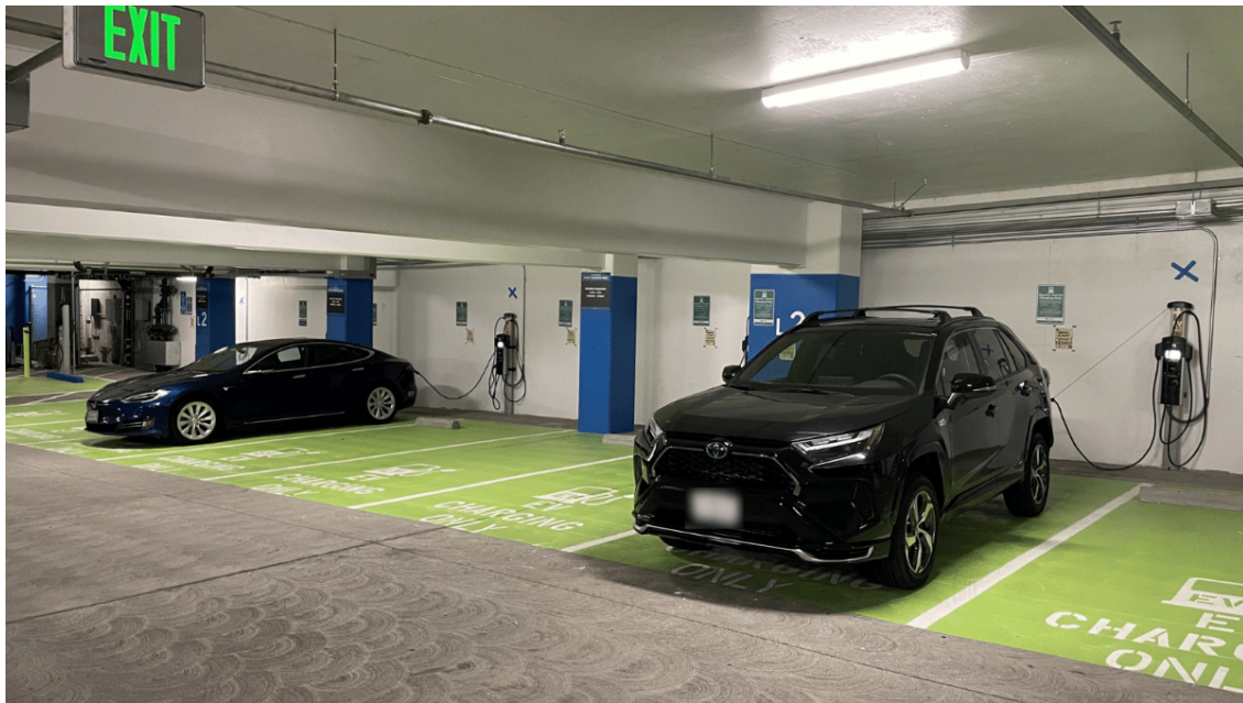
The Pasteur Staff Garage features 12 EV charging ports at the lower level 2 (L2) of the garage.
