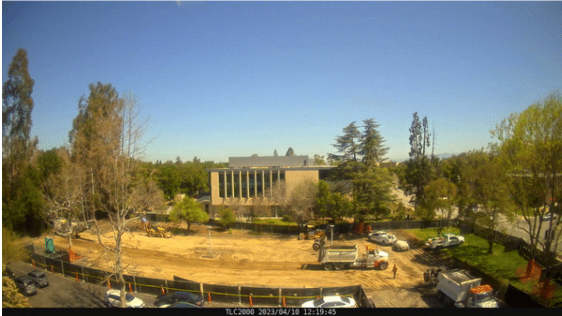
Timelapse of the Blake Wilbur Drive roadway extension project on April 10, 2023
