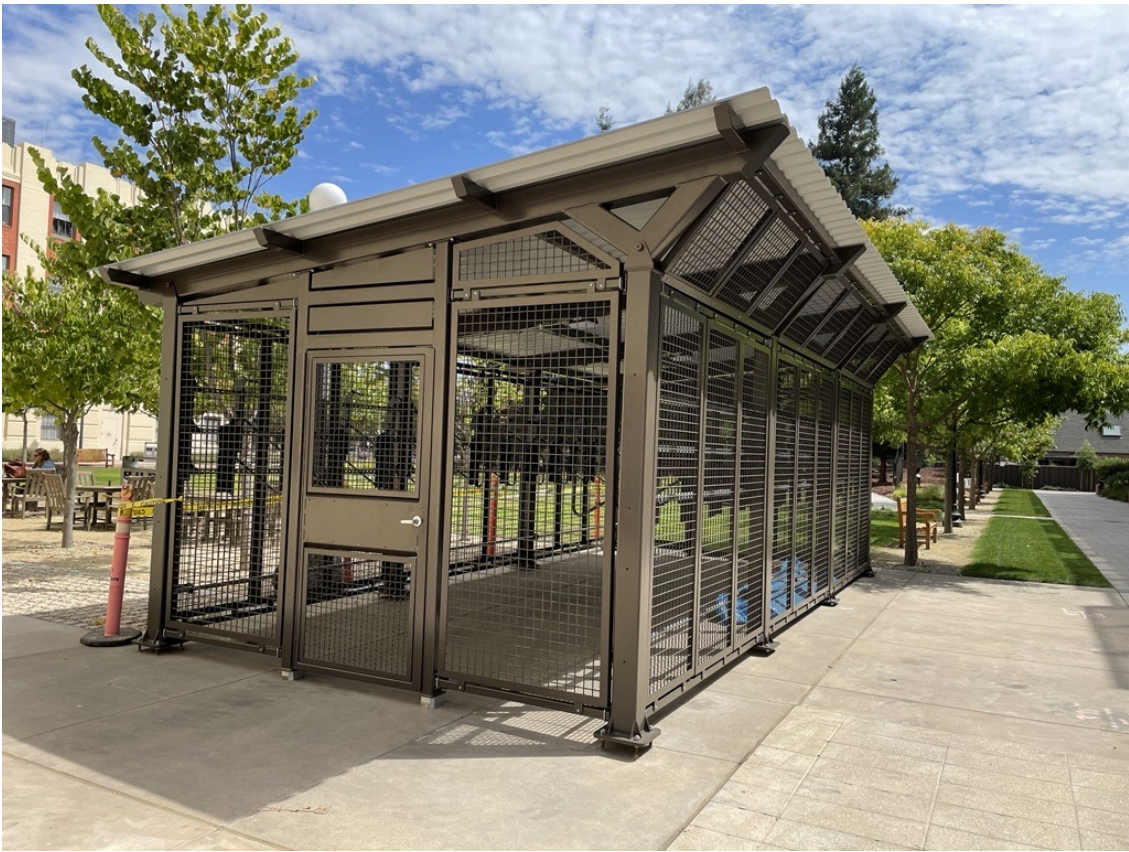
The Hoover Pavilion bicycle cage installation is in progress
