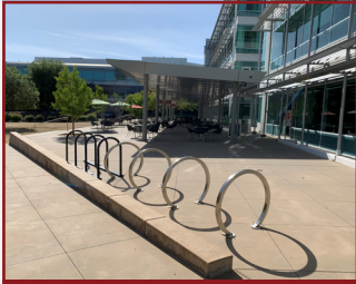
Pavilion C & D Bike Racks
